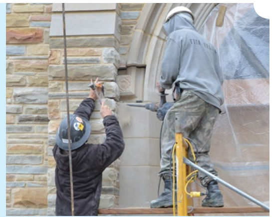
Workers carefully set the decorative limestone pieces.
