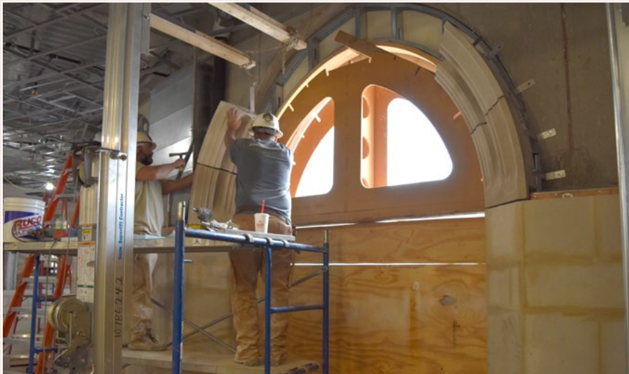
Workers carefully position and set the massive limestone archway components.
