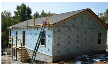
5 Church Streeters helped this past Saturday building walls and shingling!
